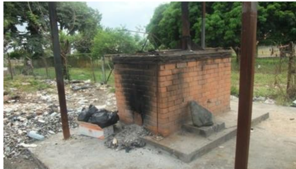
Figure 10: The current incinerator
